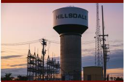
Reconditioning of the industrial water tower in Hillsdale's Manufacturing and Technology Park began in June. Both the interior and the exterior of the water tower were extensively cleaned and repainted. These are the first major repairs since it was constructed in 1995. The work was completed in late July and the water tower has since been refilled and returned to service.
