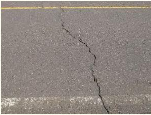
Transverse cracking
