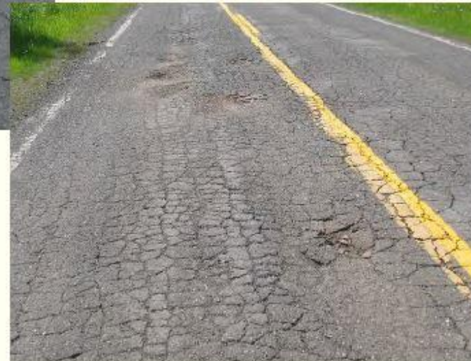
Alligator Cracking
