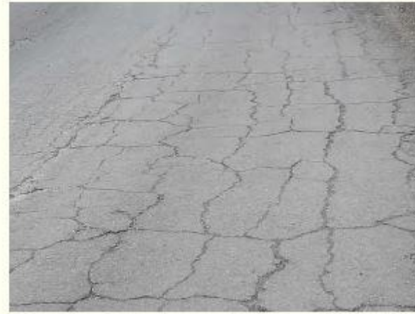
Block cracking
