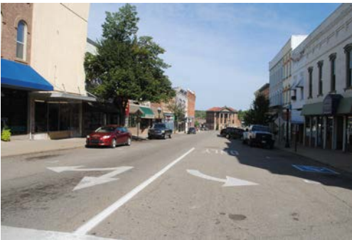
HOWELL STREET One lane from Broad to McCollum Streets. One-way road with angle and parallel parking on one side, parallel parking on the other and an additional left turn lane. Road width averages 45'. Building face to building face dimensions avg. 70'.
