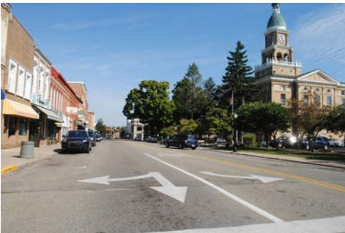
HOWELL STREET Two lane at McCollum Street,, with a right turn lane, two-way road with parallel parking on both sides. Road width averages 50'. Building face to building face dimensions avg. 80'
