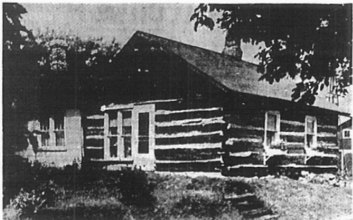
Conversion of schoolhouses into homes is not a present-day development inspired by school district consolidations, although the movement has been accelerated thereby. Shown above is a log school built sometime before 1870 near Lickley's Corners. In 1910 it was moved to the Richard Loney farm and in 1926 to its present location two miles from where it began life as the Elm School. Now owned by Mr. and Mrs. Noah Glendening, it has been modernized as is evident in the picture. Needless to say it is a landmark in that section of Hillsdale County.
