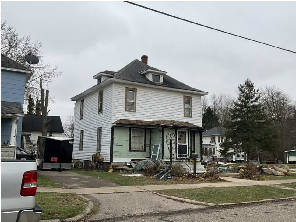
54 WESTWOOD ST 2024-12-17 BUILDING PER
